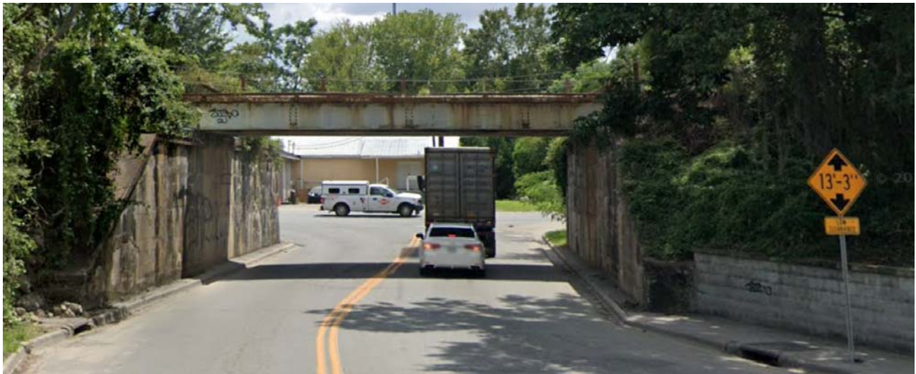
FIGURE 4.2 VERTICAL CLEARANCE AT E. LATHROP AVENUE
