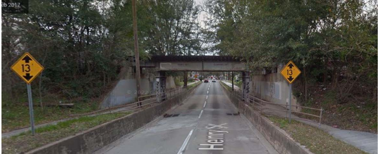
FIGURE 4.3 VERTICAL CLEARANCE AT EAST HENRY STREET
